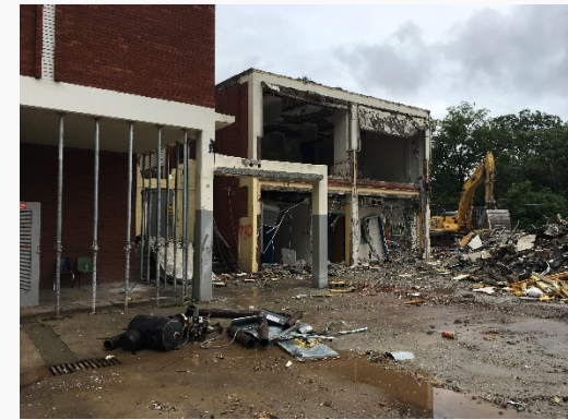
Reshoring of failing existing column
